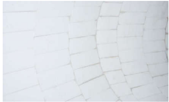
Wedge Type Liner Fitment (Alumina Bend)
